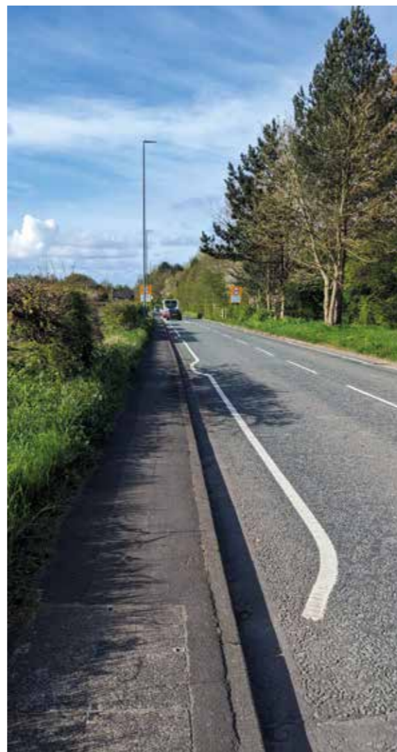
Figure 5.1 Narrow footway in Knowsley Village
